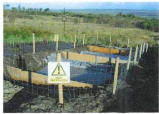
COMPLETED SETTLEMENT POND SYSTEM SCALE NTS
